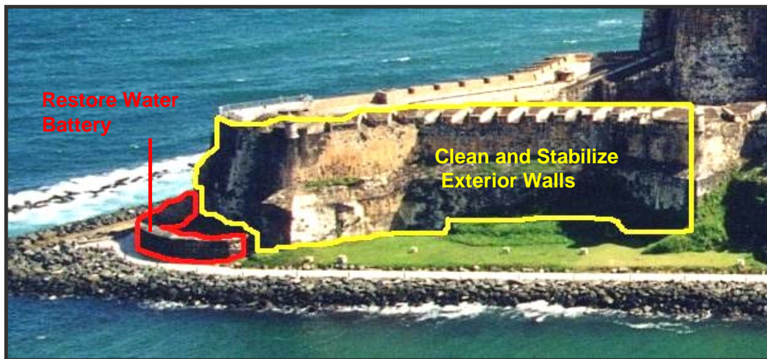
El Morro Water Battery and walls to be restored. The existing Promenade (“Paseo”) is shown in the foreground.
