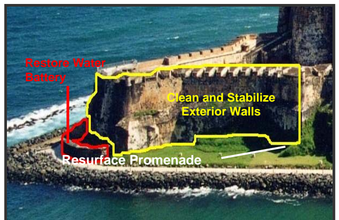
Restoration projects at El Morro
